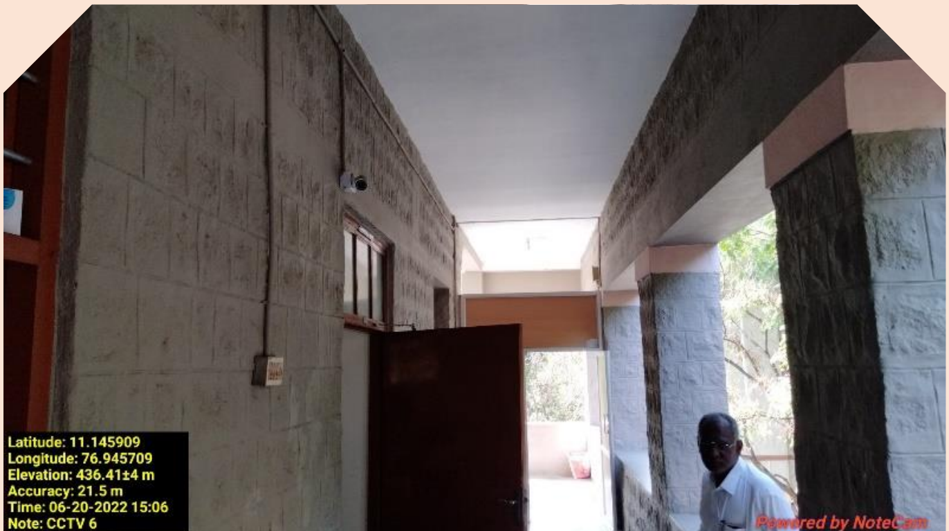
CCTV at Office Veranda
